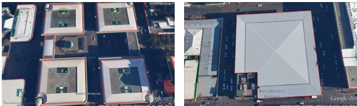
Figure 23: Colour-coded rooftop area measurements.
