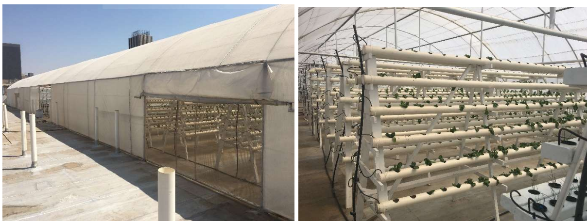
Figure 4-19: Massive hydroponics setup above the Greatermans building. Source: (Author)
