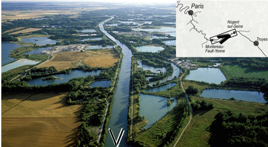
Fig. 6 Aerial photograph of the Bassée floodplain, upstream of the Seine-Yonne confluence, showing the multiple sandpits, generally filled by groundwaters, and the straightened, deepened and dredged navigation channel with its levees and dikes. A former river meander part, now a disconnected water body, is visible on the right centre of the picture. Only patches of the original riparian forest remain between the sandpits and the agricultural areas [© La Pérouse 2005]
